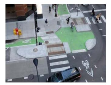
Figure 3.30. Example of protected intersection. **Source**: **Toole Design Group**
