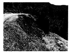
may also require full road closure. Inboard retreat does not appear feasible due to steep inboard slopes, hard rock, or alignment issues.
