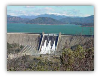
thick at the top. Shasta Dam is a curved concrete gravity-type dam with 6.5 million cubic yards of concrete weighing 15 million tons.
