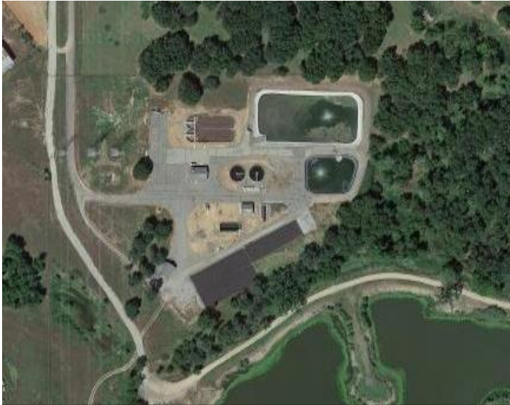
Photo 1: Wastewater Treatment Plant
