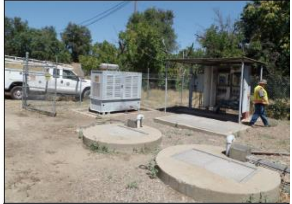
Photo 2: Main Lift Station
